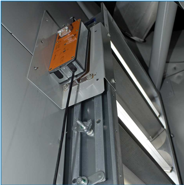
Actuator for modulating air inlet dampers
