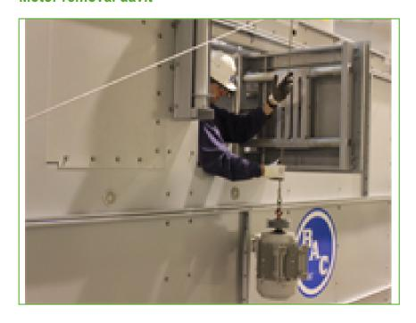
With the motor removal davit, the motor <a href="mailto:can easily be lowered">can easily be lowered</a> from or lifted to the motor base without the need for extra heavy material of scaffolding.
