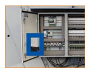
Protects electronic components in the electrical panel during extremely cold temperatures.
