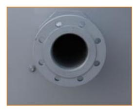
Flanges facilitate piping connections on-site.
