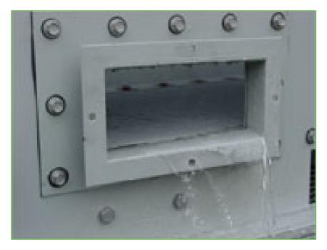
A factory-installed clean out port
