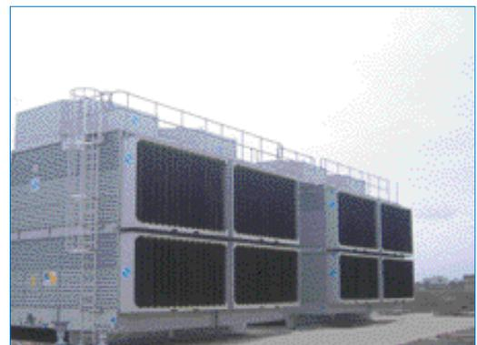
Figure 11: Intake and discharge sound attenuation on a BAC Axial Fan Open Cooling Tower
