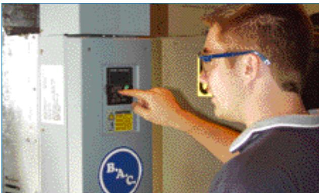
Figure 8: VFD with Integrated Bypass
