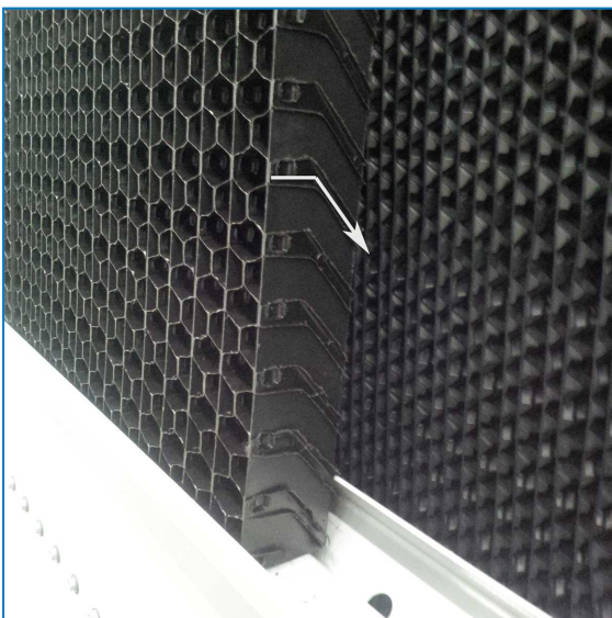
Orientation of the combined inlet shield
