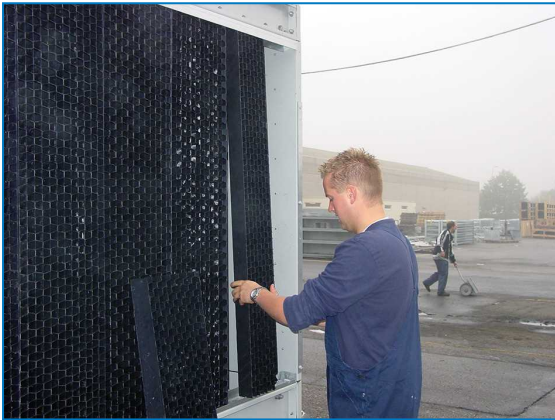
Remove combined inlet shields
