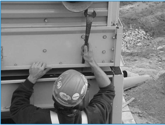
Corner alignment with drift pin
